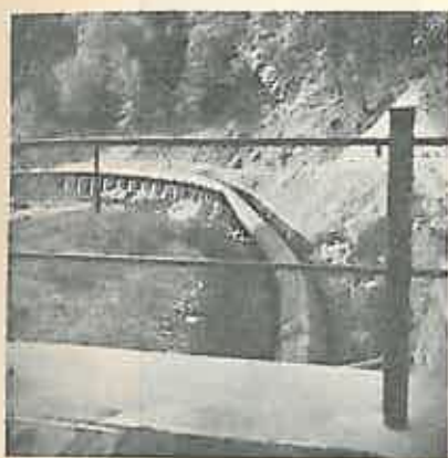
Fig. No. 4. — Conducta pleacă dela baraj.
